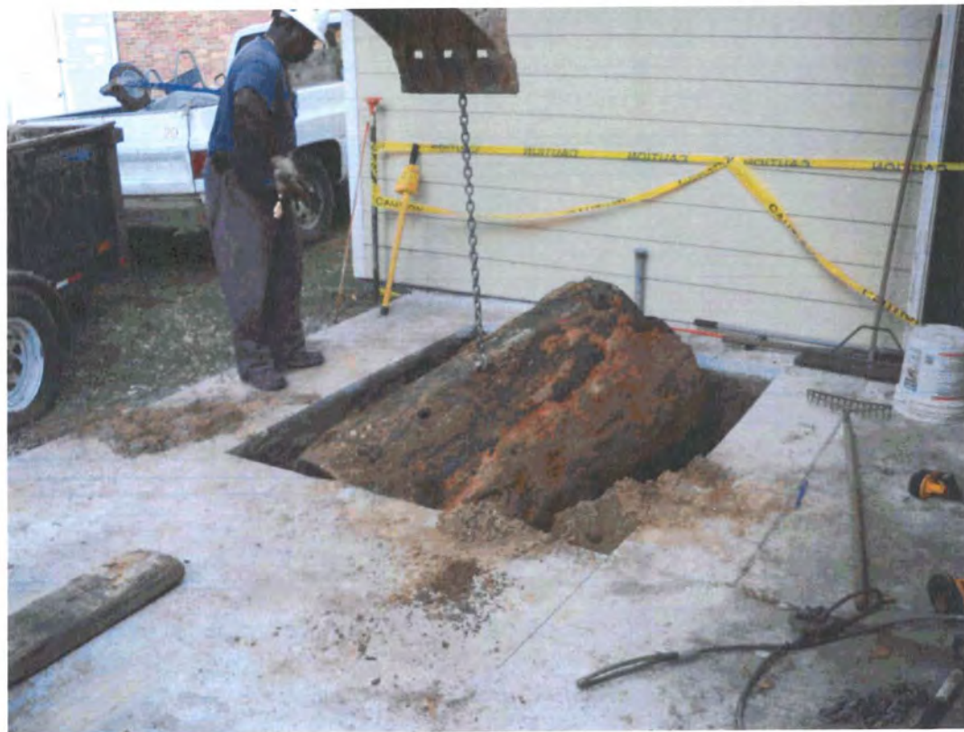
Picture 2: UST 322Ash-1 extraction in progress.
